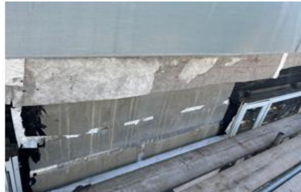
A photo showing Phase 2 North Elevation – Existing cladding removal works complete
