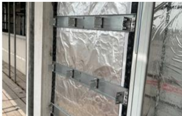
A photo showing Phase 1 South Elevation – Helping hand bracket installation works progressing
